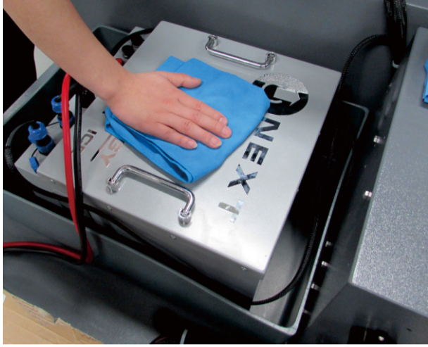
Clean Stains on Top of Battery
